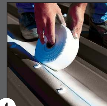
4 Reinforce existing seams with Spunflex® or Butyl Tape and base coat.
