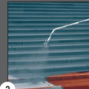
2 Prime with Conklin Encase® Metal Primer.
