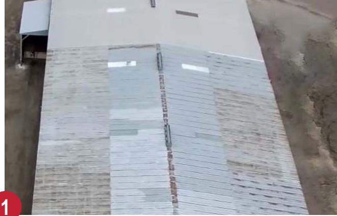
Rusty metal roof prior to restoration work.
