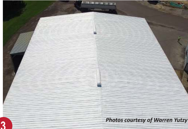
Metal roof after Benchmark® acrylic top coat.
